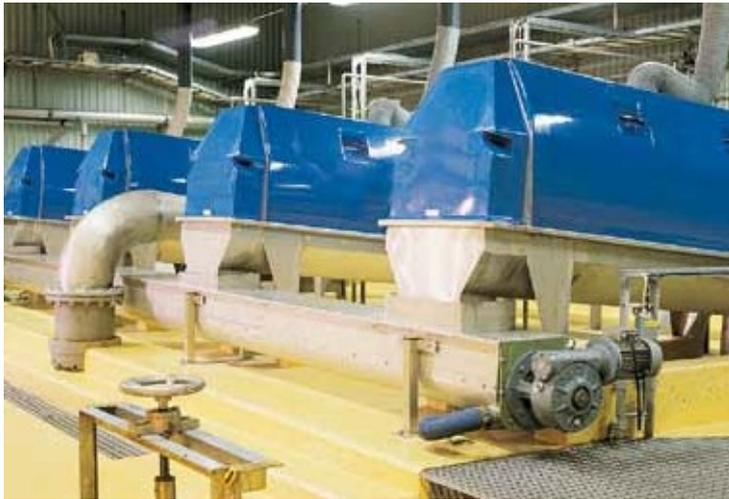
*Roto-Sieve drum screens, model RS-51, installed at Kullavik treatment works in Kungsbacka.*
